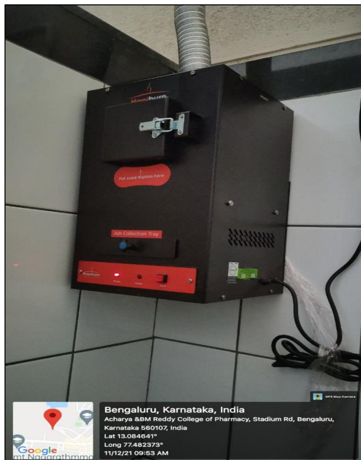
Sanitary Napkin Incinerator installation at women's rest rooms
