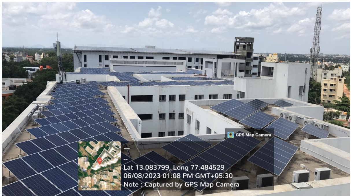
Photos of Solar Panels
